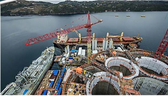
Iron ore bulk carrier (top) and fly ash bulk carrier (left) moored at the flotilla for installation of solid ballast in the Gravity Based Structure.
