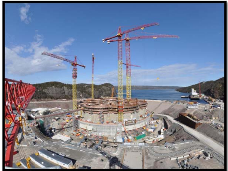
Gravity Base Structure - May 2014
