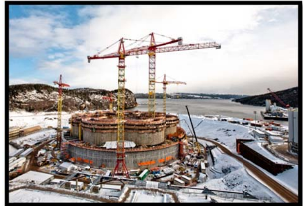
GBS cantilever walls (bottom perimeter walls) - December 2013
